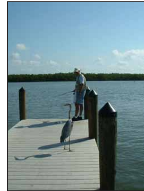
View of Estero Bay from the newly reconstructed dock.
