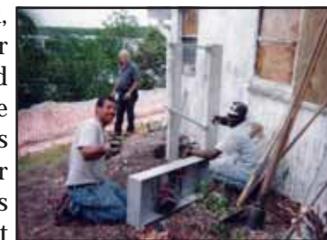
Luis Ortiz and Jeanty Joseph install the new electrical panel at the back of the Mound House garage as Tom McLean looks on.
